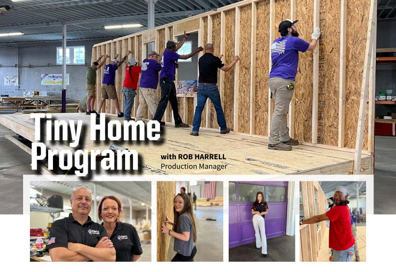
Veteran Tiny Homes are modular homes built at the PHH headquarters in our manufacturing warehouse. These modular homes are built just like any traditional stick-built house. They are delivered to sites and placed on crawl space foundations. Our current builds are 320 sq. ft. (10 ft. x 32 ft.) and come equipped with a full-size refrigerator, stove, microwave, stacked washer and dryer, and a small heating and air unit.
